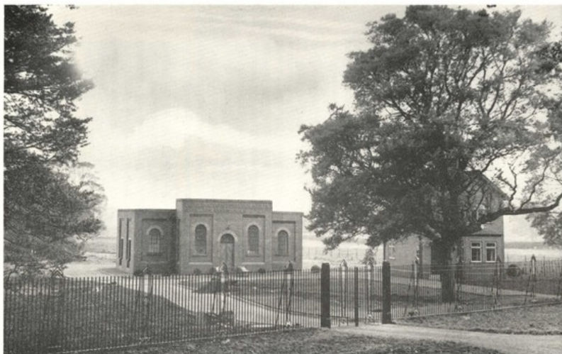
A General View of the Burton Agnes Pumping Station and Attendant's House.
