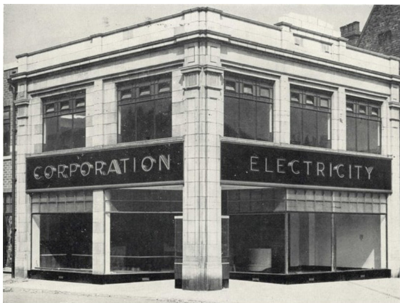
NEW ADMINISTRATIVE OFFICES AND SHOWROOM ELECTRICITY DEPARTMENT.
